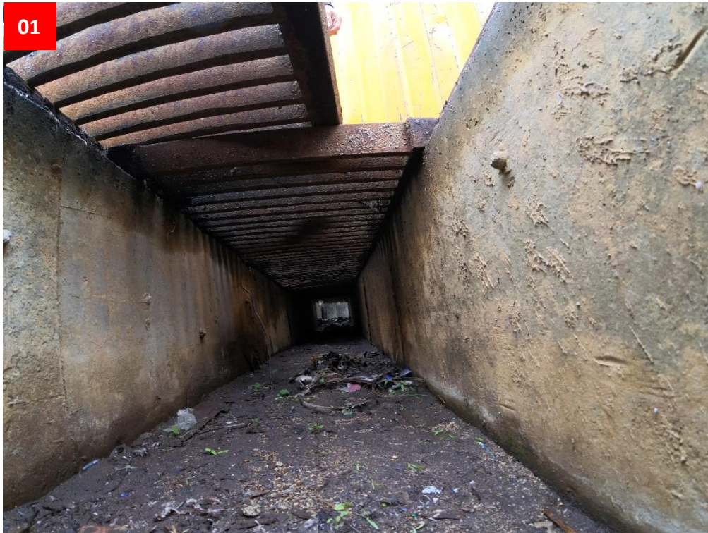
b) Site photo taken on 3.3.2026
